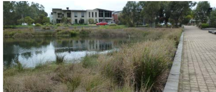
Figure 3-5. Lochiel Park MAR wetland is integrated into the development's water-sensitive urban design
