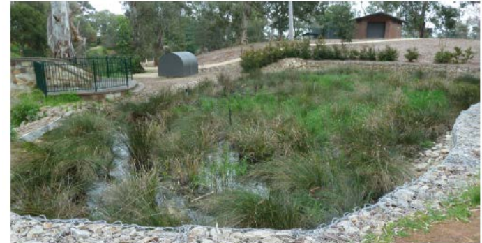
Figure 3-3. Ridge Park vertical biofiltration bed: Water is pumped from the creek and is filtered as it percolates through the wetland bed. An injection well is contained in the grey-domed box.
