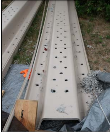
Bulkhead sheet perforated belowground
