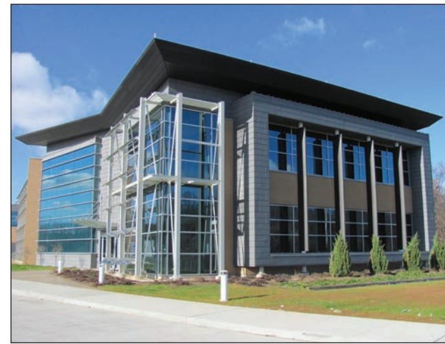
The Advanced Energy Center at Stony Brook University
